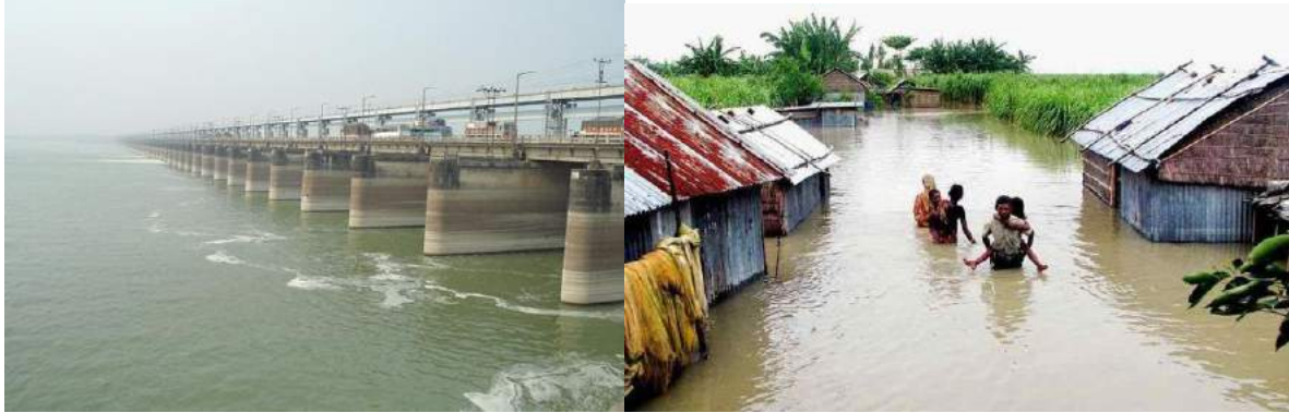
Farakka Barrage. Photo: Google; Flood affected people in Kushtia due to open all sluice gated of Farakka barrage. Photo: Bangla Tribune
